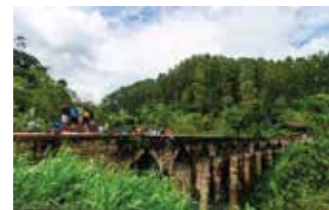
Nine Arch Bridge (90m)
